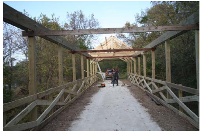
Building a covered bridge on the Blue River Trail.
