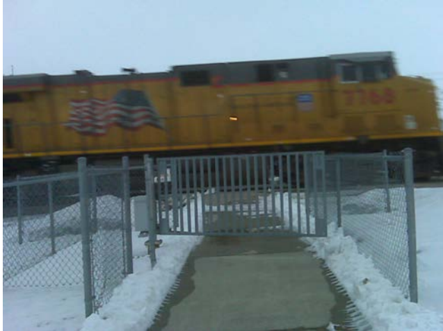
Train activated safety gate, Waterloo, NE
